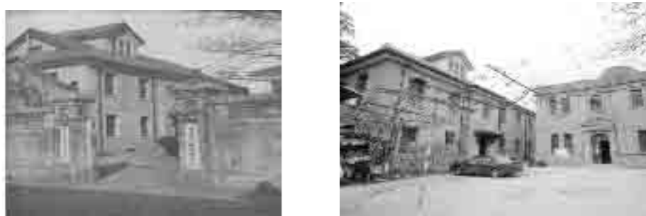
Fig. 6 The Geological survey in 1931 Fig. 7 Two German style buildings of Bingmasi yard in 1996
